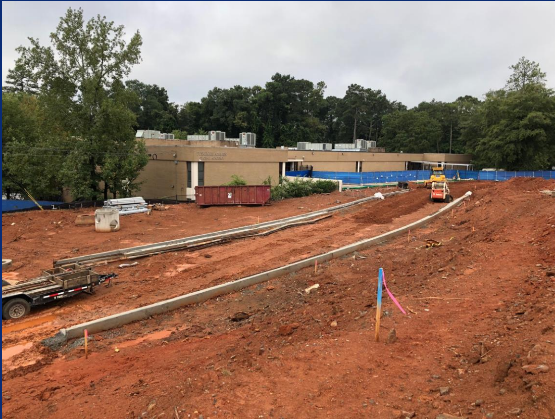
Curb and Gutter Concrete Poured at New Richland Road
